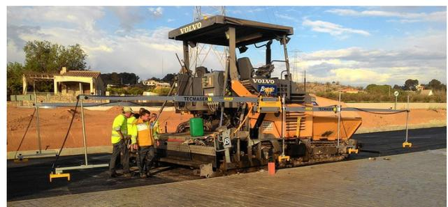
Figure 1: The Big Sonic-Ski from Moba with four CAN-connected sensors for asphalt paving (Source: Moba)
