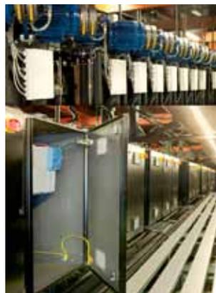
Figure 3: The safe control solution includes customized enclosures for each of the more than one hundred drives in the upper and lower machinery
