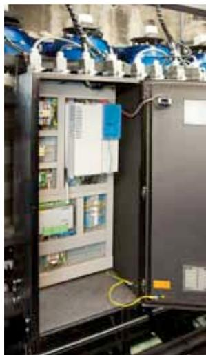
Figure 1: Each enclosure contains one ICU computer by Unican (bottom left) and an SK 535 frequency inverter by Nord (top right)
