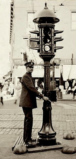
On August 5, 1914, the American Traffic Signal company installed an electrical traffic signal system on the corner of East 105<sup>th</sup> Street and Euclid Avenue in Cleveland, Ohio. It had two colors, red and green, and a buzzer, based on the design of James Hoge. The design allowed police and fire stations to control the signals in case of emergency.
